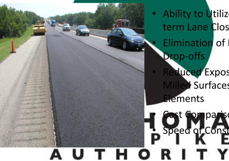
• Ability to Utilize Shortterm Lane Closures **Elimination** of Edge Drop-offs Reduced Exposure of Milled Surfaces to
